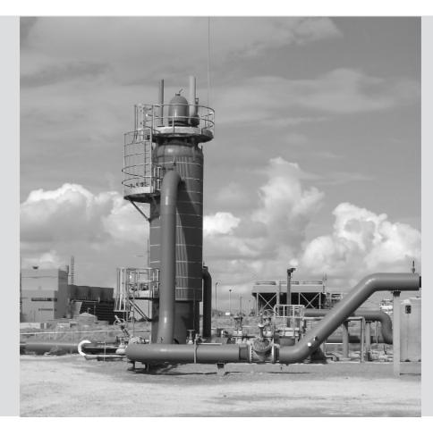
Blundell geothermal power plant near Milford, UT, USA. This 38-MW plant consists of two generating units powered by geothermal steam. Steam is created from water heated by magma at depths up to 6100 meters below Earth's surface. (Courtesy of PacifiCorp.)
